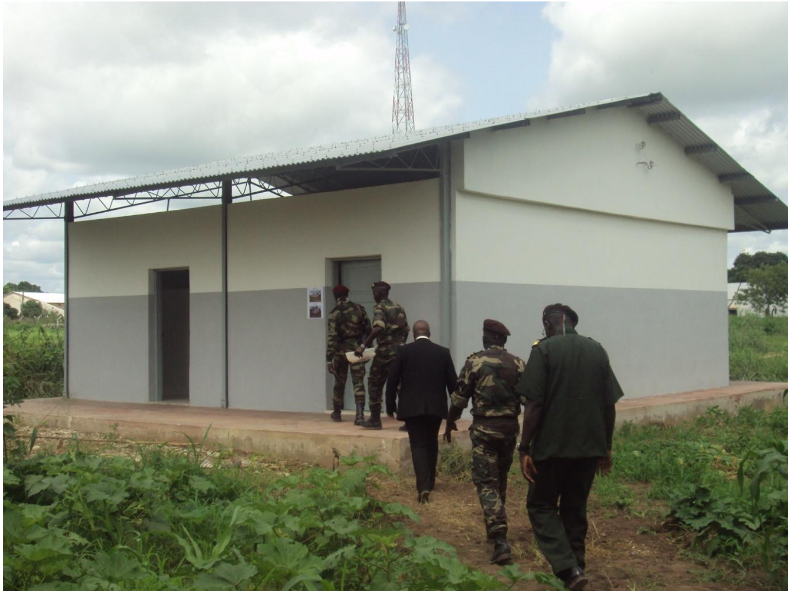
Figure 2 - Military building rehabilitated in Gabu barrack. - - Handover ceremony August 10, 2011
