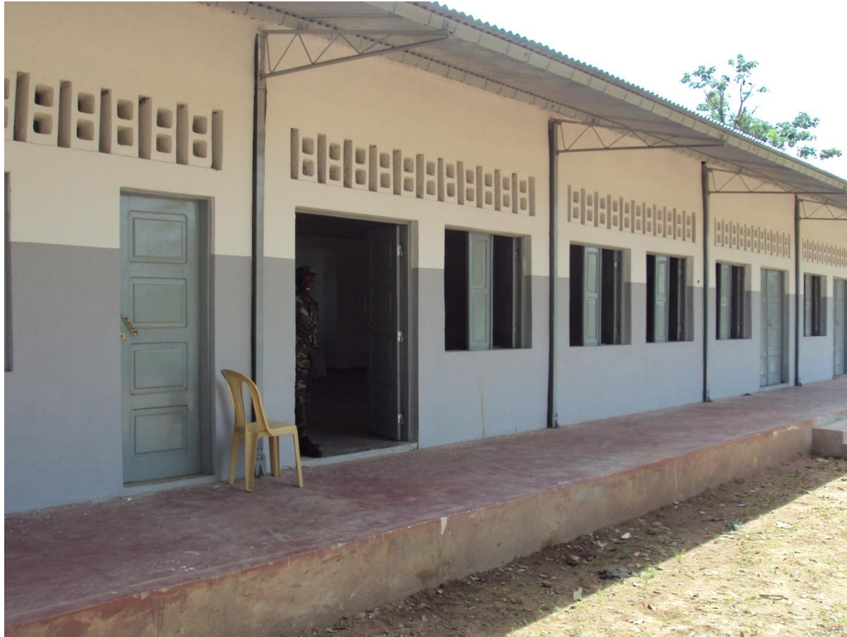
Figure 3 - Military building rehabilitated in Gabu barrack. - - Handover ceremony August 10, 2011
