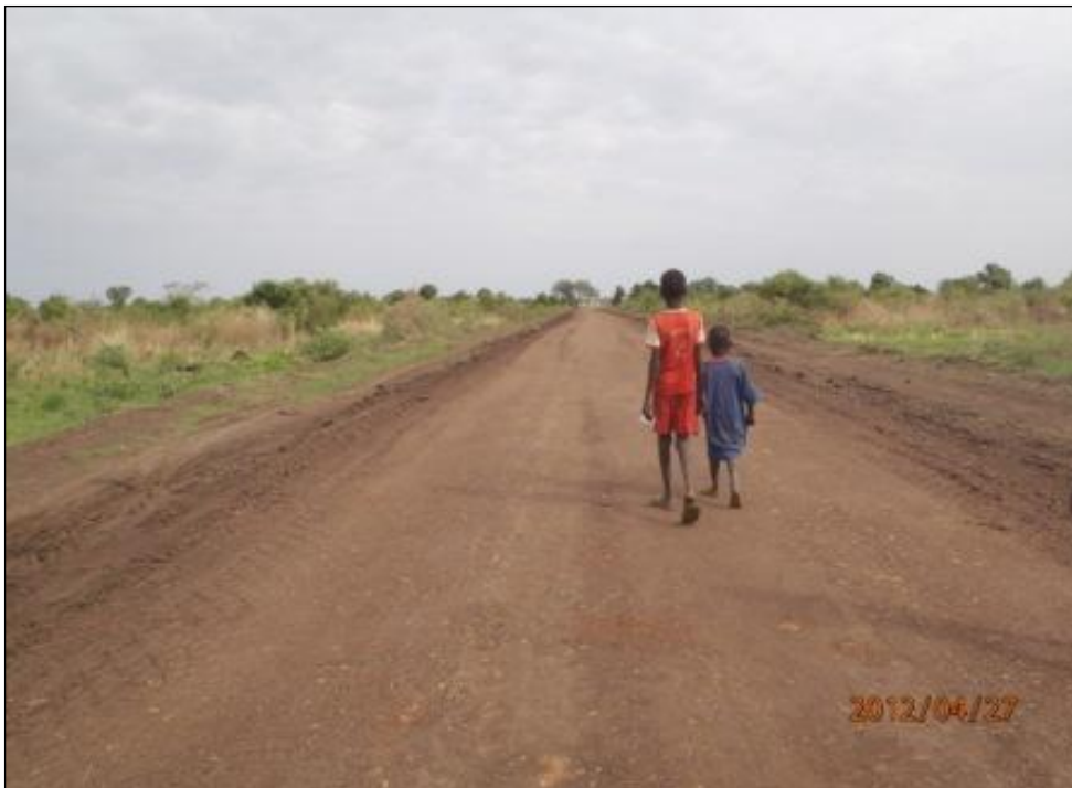
Package 2 – Gravel wearing course on the 60KM Akobo- Pochalla Road
