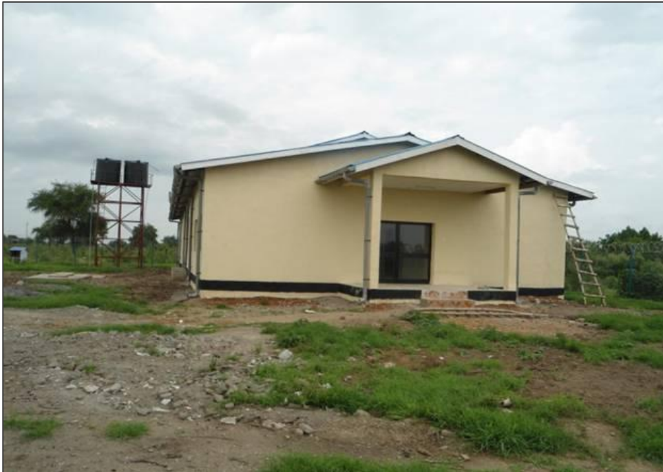
Construction of Radio Station in Bor, Jonglei State
