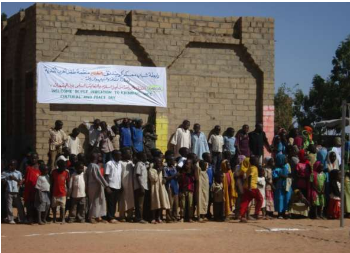
One of the 20 schools constructed by War Child Canada in West Darfur using stabilized soil blocks, an environmentally sustainable alternative to kiln-fired bricks.
