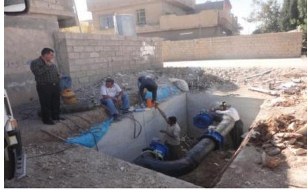
Construction of valve chamber for Sarchinar trunk pipes
