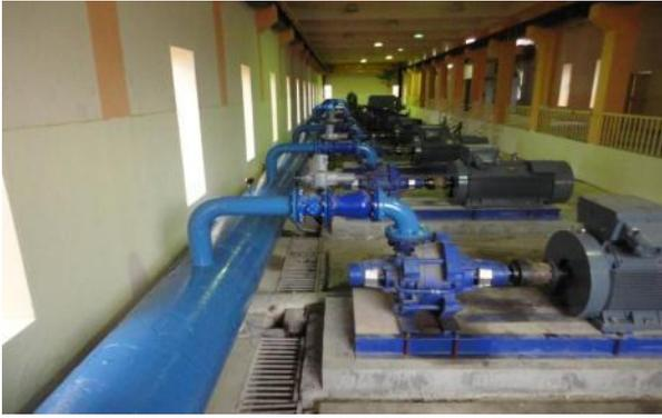
Installation of variable speed pumps in Sarchinar water project
