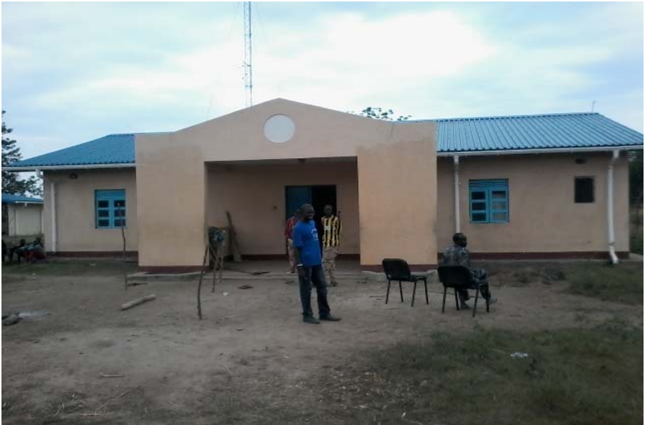
Makuac police station, 2014
