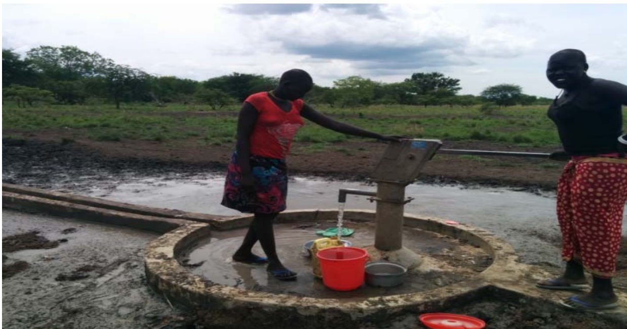
Human water access points (borehole) constructed at Aburiri, 2014
