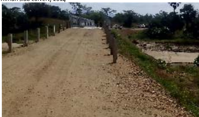
Approaching view of Kidepo Bridge, 2014
