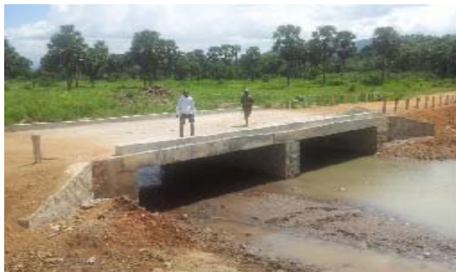
Kimam slab culvert, 2014
