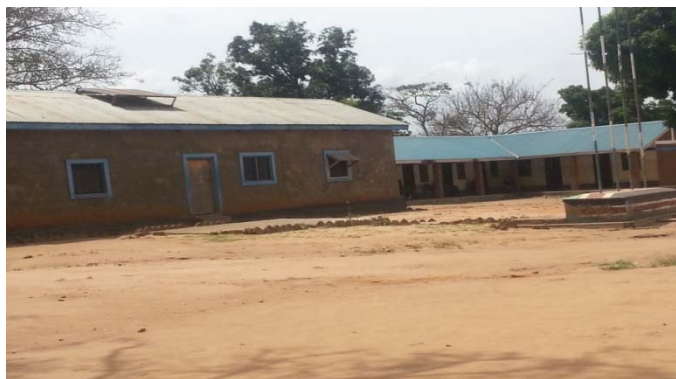
The former (used before) Magwi CHQ, 2014
