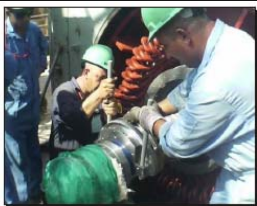
Taji: Installation of procured equipment
