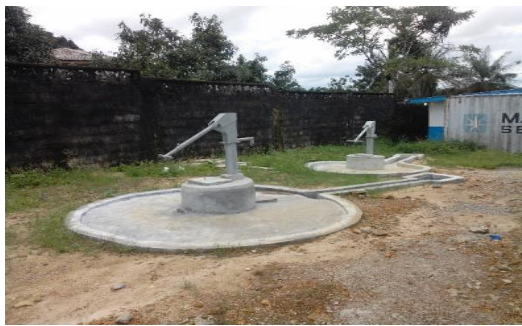
Two newly constructed hand pumps at the hospital
