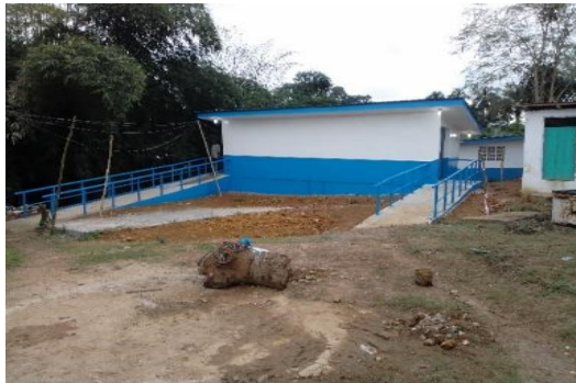
6 cubical latrines construction in the compounds of the Hospital
