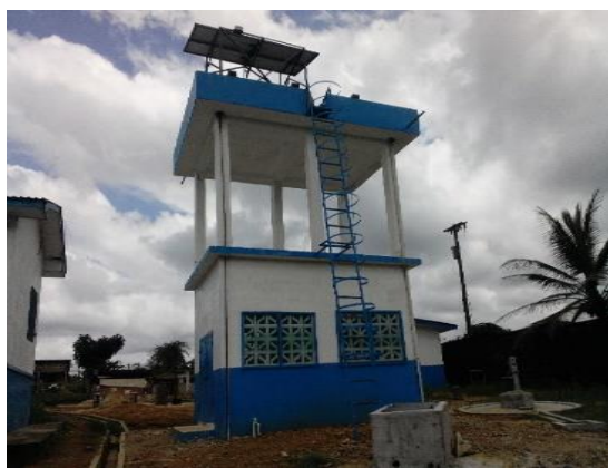
Above: Newly Constructed Water tower, which did not exist prior to project
