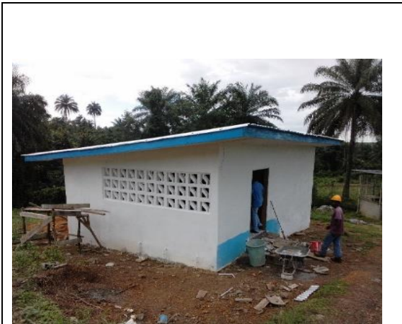
Above: the newly constructed laundry at hospital
