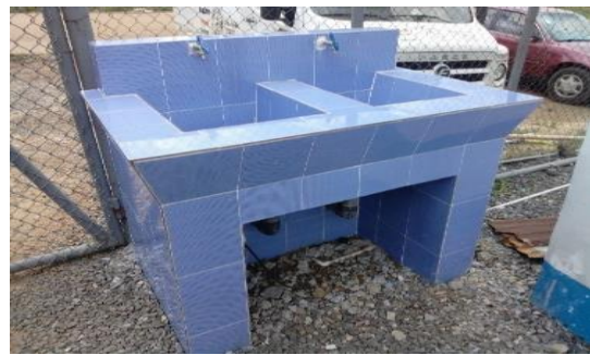
Above: Hand washing stand at hospital
