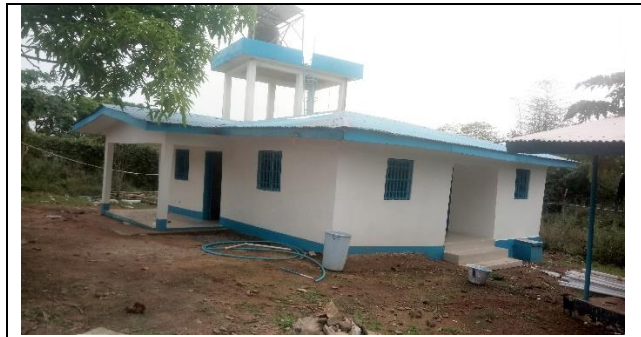
Constructed Maternal waiting home in Nyehn
