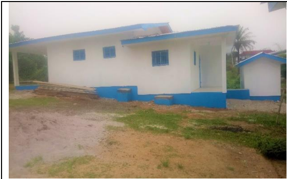
Constructed Maternal waiting home in Bensonville
