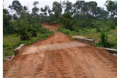
Construction bridge (dalot) in Moata –Démou II (Forest Guinea).
