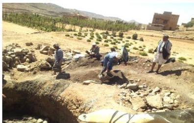
One of the requirements was also to build check dams and excavate ponds in the valley to harvest rainwater so the nearby shallow wells would later absorb the water. These works revived eight shallow wells and the water level started increasing gradually. Almost three hundred families benefited from the water of shallow wells and 13 hectares of land were recovered for agricultural use.
