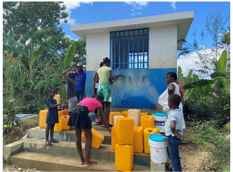
Water Distribution point
