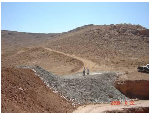
Spillway of Hafir No.8
