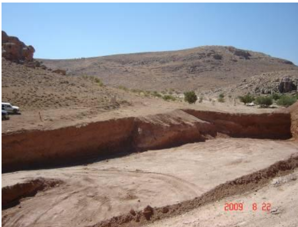
Excavations in Hafir No.8
