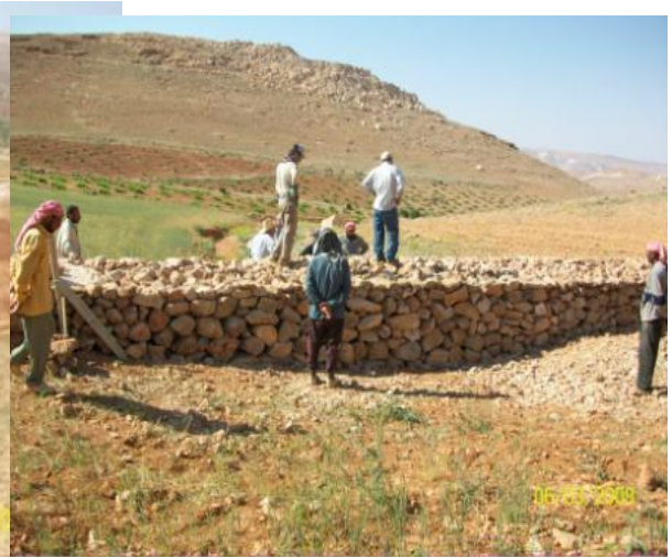
Construction of more check dams
