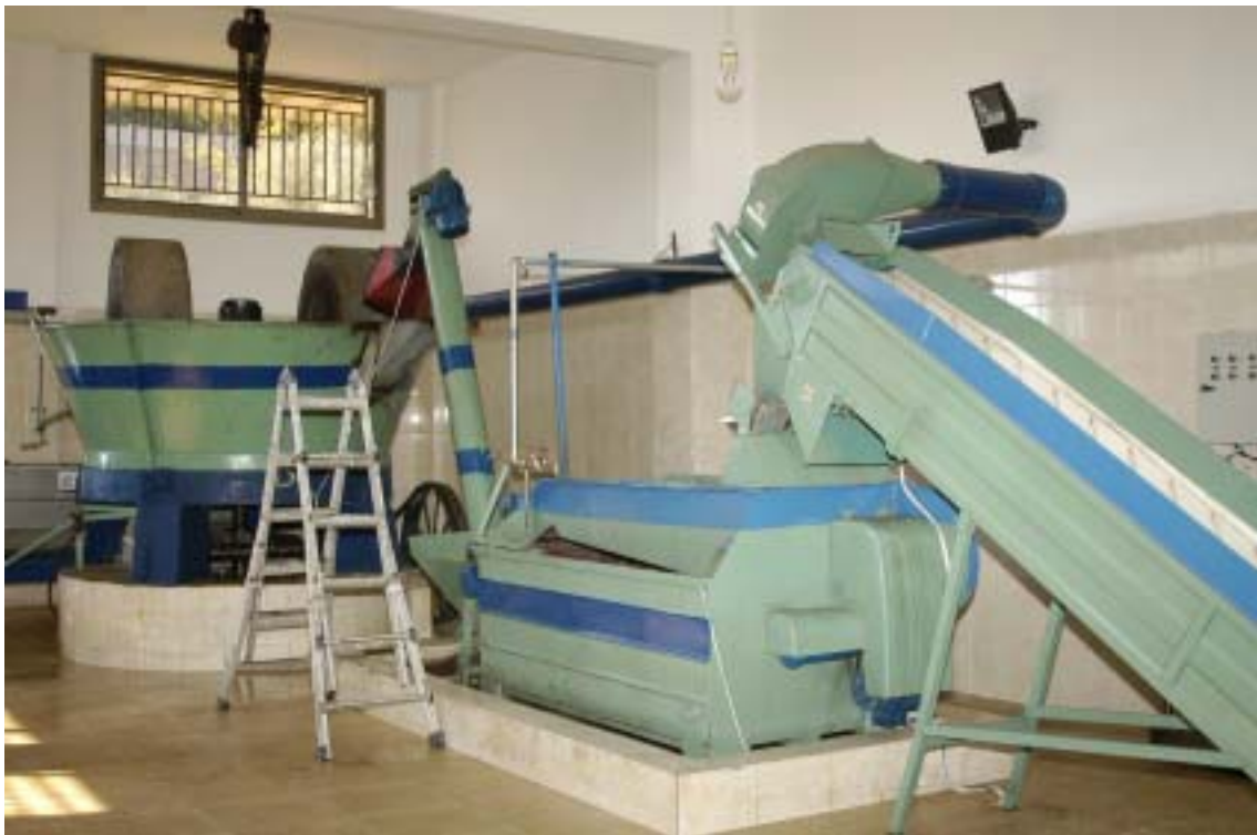
Rehabilitation of olive oil enterprise and provision of equipment, Khiam
