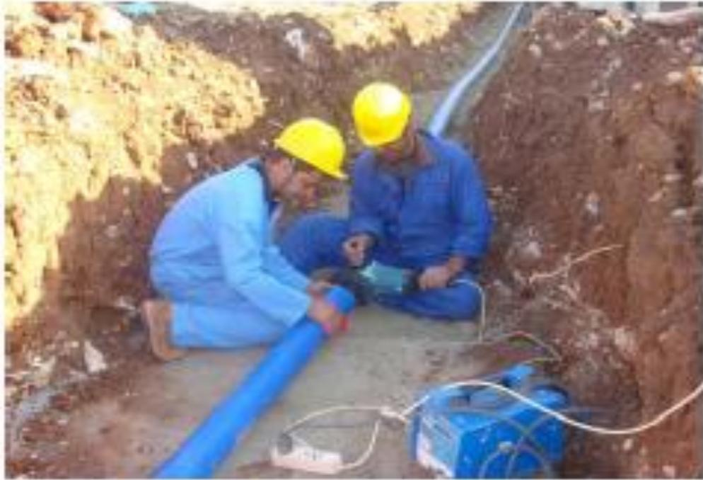
**Laborers Jointing the PE Pipes Using Electrofusin Technology**
