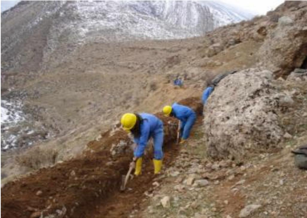
**Excavations for Laying of Pipeline**
