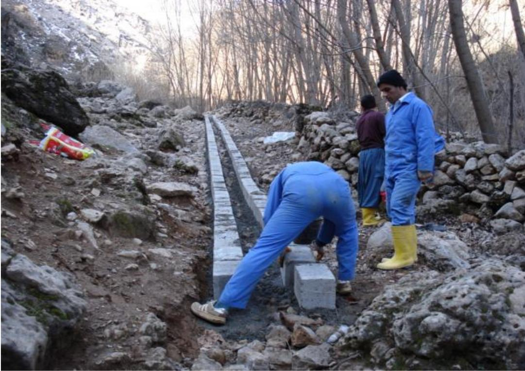
**Construction of Sidewalls to Lay Pipeline on the Rock Bed from Source to Water Tank**
