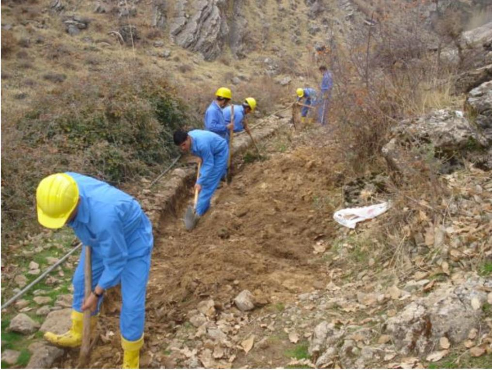
**Excavations for Laying of Pipeline**
