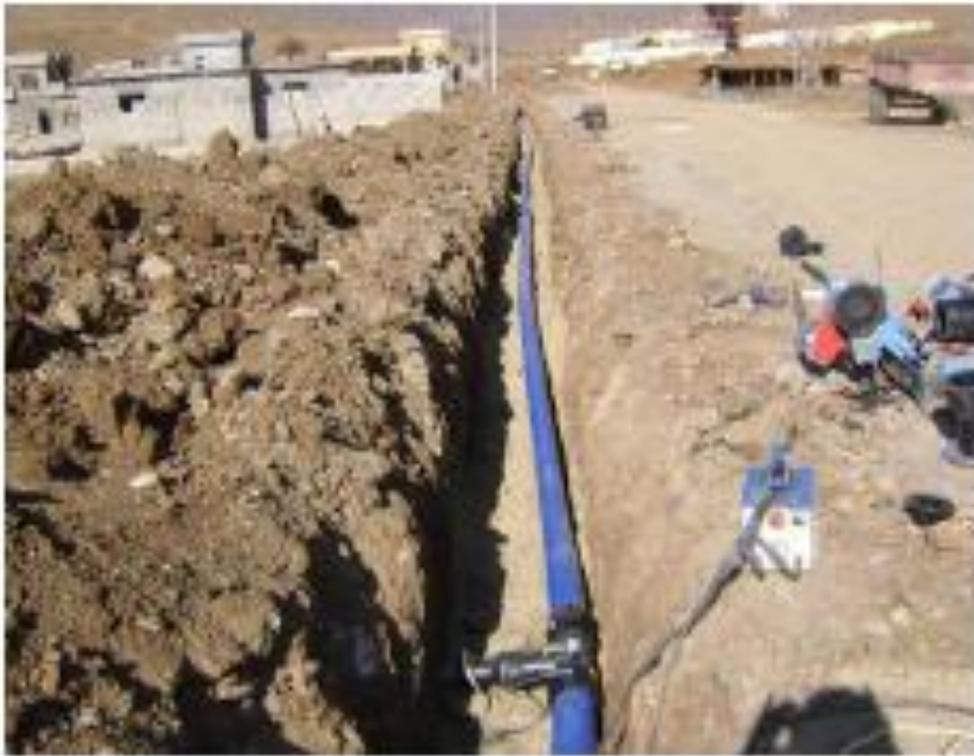
**Joining of PE Pipes using Electrofusion Joining Technology**
