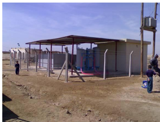
View of another rehabilitated Compact Unit in Al Gasaba, Wassit governorate
