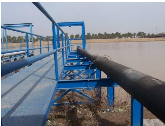
Newly constructed Intake structure – Al Sadr Compact Unit, Missan
