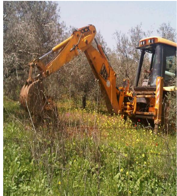
Figure 3: Excavating an inspection pit in Blat
