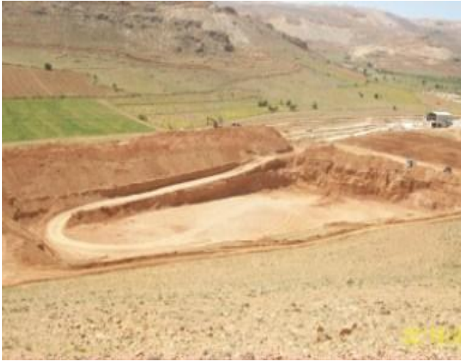
Completion of Hafir No. 7
