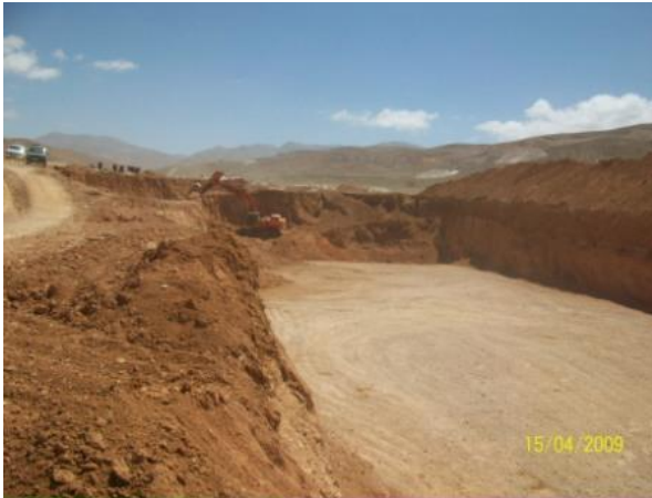
Excavations in Hafir No.11
