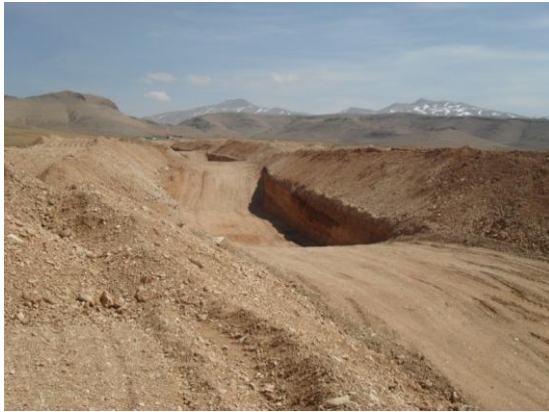
Excavation works of reservoir RR12
