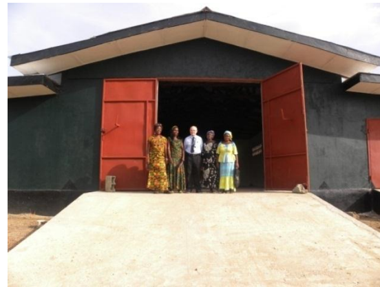
Palala Warehouse (Bong)
