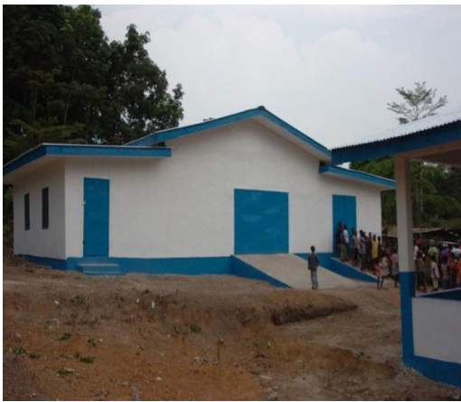
Yanewoun Warehouse (Bong)
