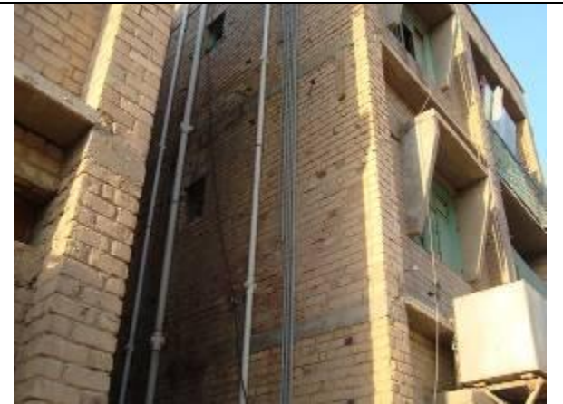
Semawa/ rehabilitation of 20 building/ RCFI/SA/H05
