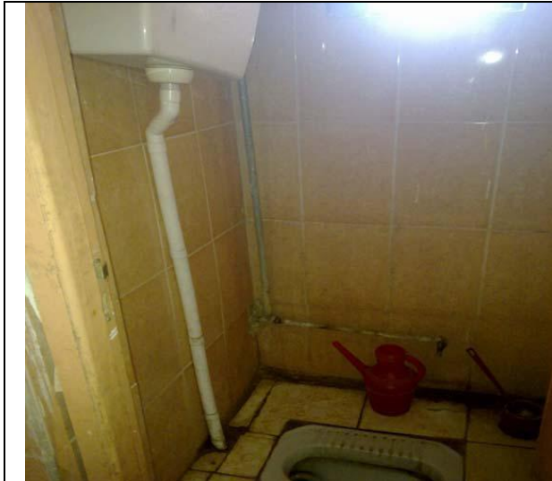
Al Faw Residential Complex / 96 flats- RCFI/BA/H02 / Basra
