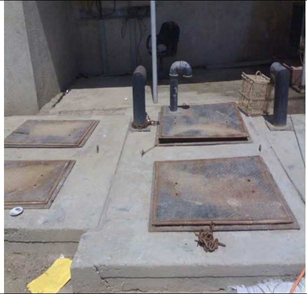
Al Faw Residential Complex / 144 flats- RCFI/BA/H05 / Basra
