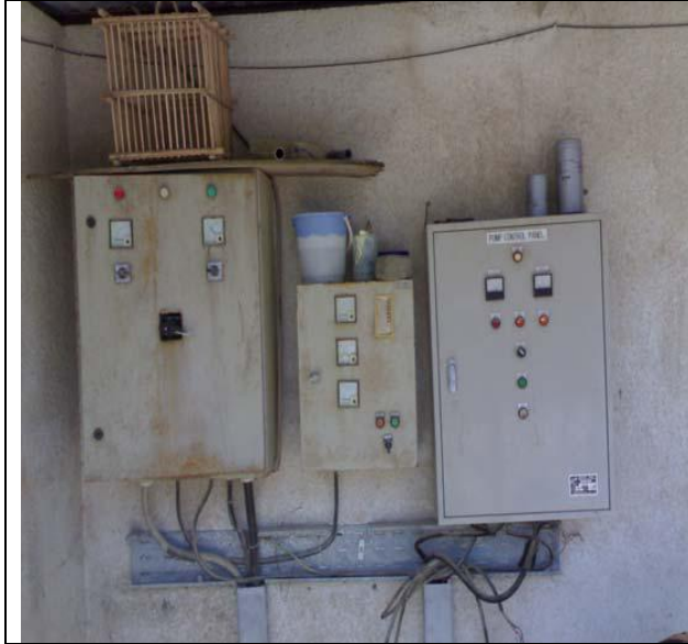
Al Faw Residential Complex / 96 flats- RCFI/BA/H02 / Basra
