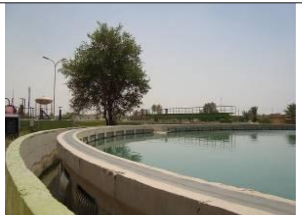
Semawa/ rehabilitation Of Rumtha WTP/ RCFI/SA/W01B
