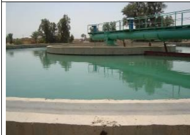
Semawa/ rehabilitation Of Rumtha WTP/ RCFI/SA/W01B
