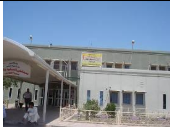
Samawa /Rehabilitation of external works /Maternity and children hospital - RCFI/SA/SDF01B
