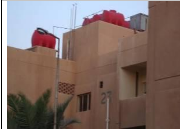
Semawa/ rehabilitation of 20 building/ RCFI/SA/H05
