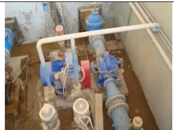
Samawa /Rehabilitation of ground water storage tanks in - RCFI/SA/W02
