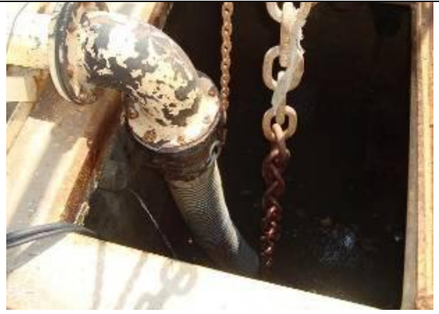
Samawa /Supply material and construct a storm water network at Al-Askri - RCFI/SA/W05
