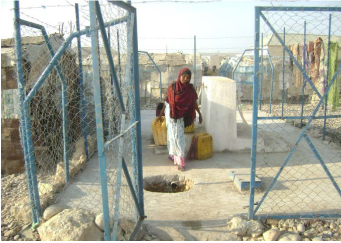
Figure 3 Newly built water kiosk in an IDP camp in Bossaso
