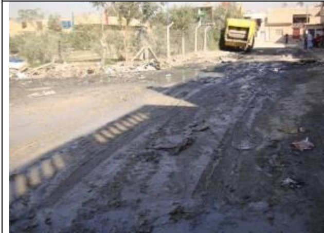
Baghdad / Rehabiliattion of garden in Sector 79/ Al Sader City / CBI activity
