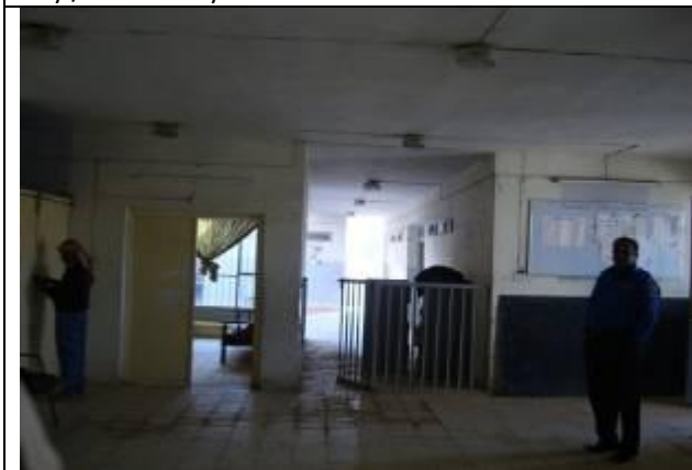
Baghdad / Rehabilitation of School in Al Entesar village / CBI activity
