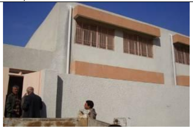
Baghdad / Rehabilitation of school / Sector 79/ Al Sader City / CBI activity
