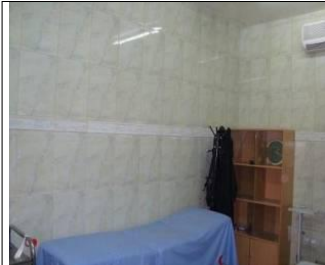
Basra / Rehabilitation & supplying of Al Baten PHCC
