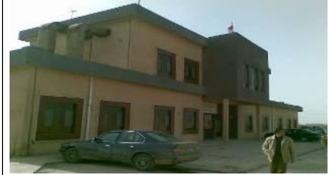
Diyala / Rehabilitation & supplying of Ba'aqwba PHCC
