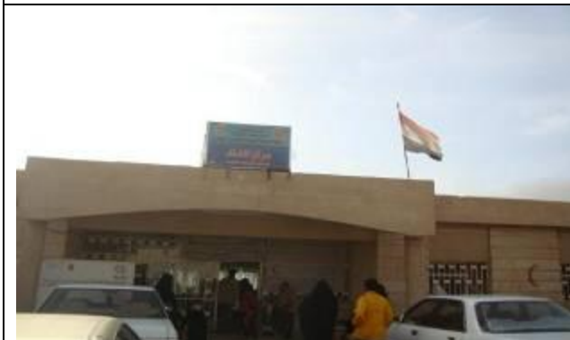
Basra / Rehabilitation & supplying of Al Shifaa PHCC
