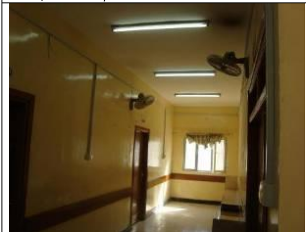
Basra / Rehabilitation & supplying of Al Baten PHCC
