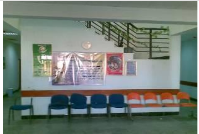
Diyala / Rehabilitation & supplying of Ba'aqwba PHCC
