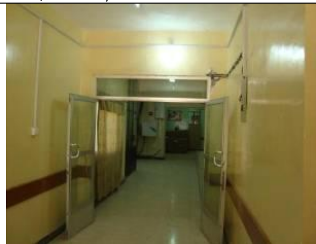
Basra / Rehabilitation & supplying of Al Baten PHCC
