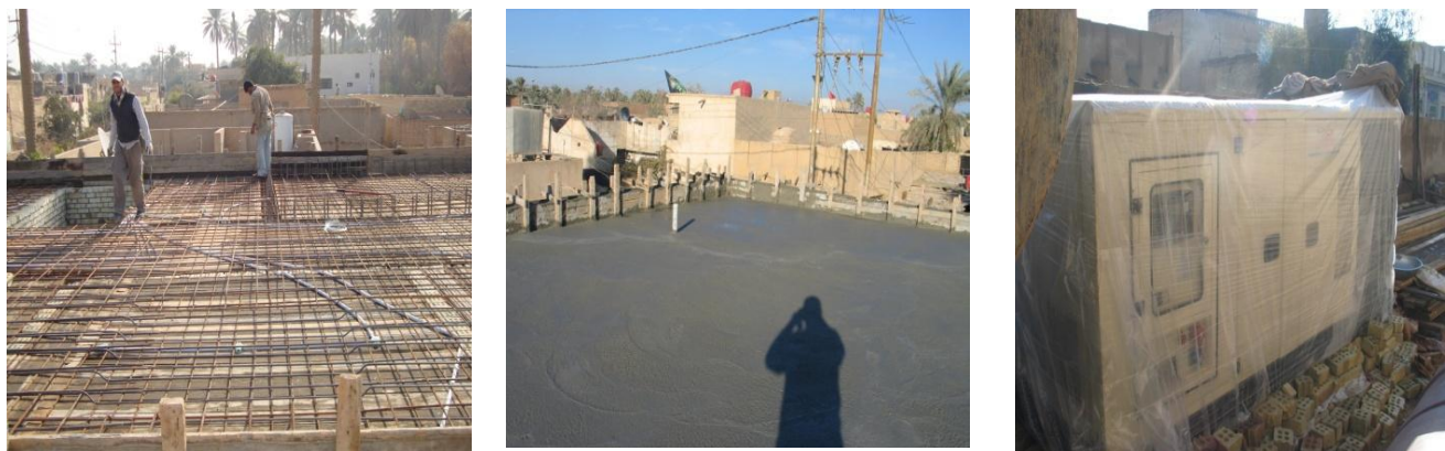
Figure 7 UNICEF engineers closely monitor & document the day to day work
