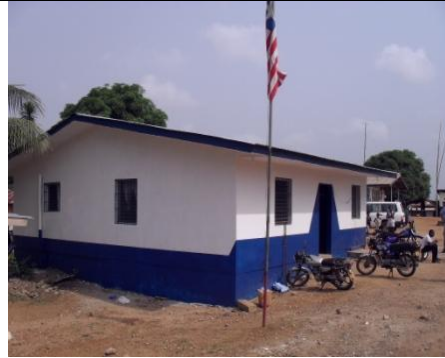
Photo 14: Newly upgraded police station in Virginia Community, Monrovia
