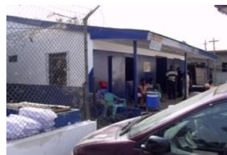
Photo 12: Newly renovated police station in New Kru Town, Monrovia
