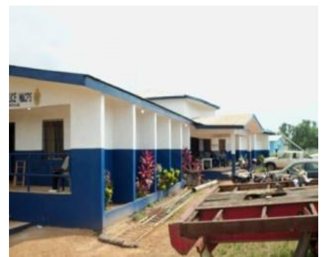
Photo 9: Newly renovated model police station in Buchanan, Grand Bassa County
