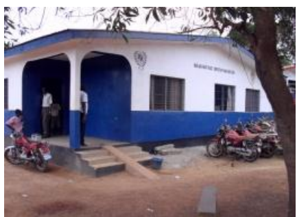
Photo 11: Renovated Police station in Ganta, Nimba county
