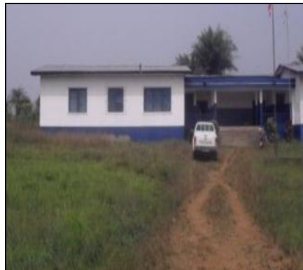
Photo 5: New renovated Police Station in Bensenville, Monsterrado county
