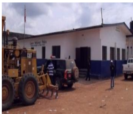
Photo 8: Kakata newly rehabilitated Model Police Station, Margibi county
