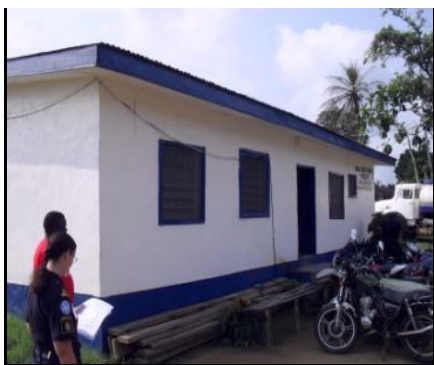
Photo 7: Salala newly renovated model police station, Bong County
