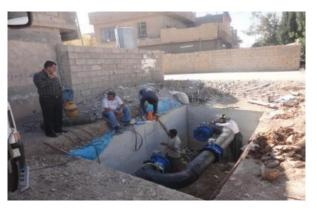
Construction of valve chamber for Sarchinar trunk pipes
