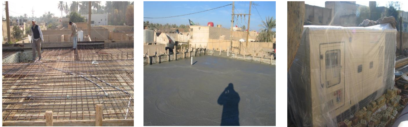
Figure 3 UNICEF engineers closely monitor & document the day to day work
