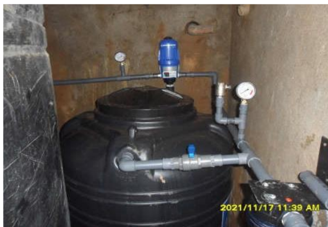
Non-electrical dosing pumps installed in water purification plant at Saliyapura Upper Division in
