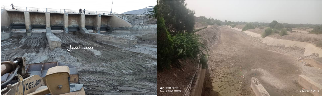
Downstream Batais dam after reconstruction of the gates, desilting and compacting
