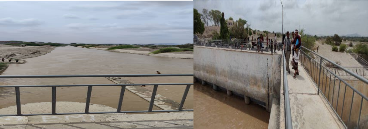
Completed work on Batais dam showing desilted channels and reconstructed gate
