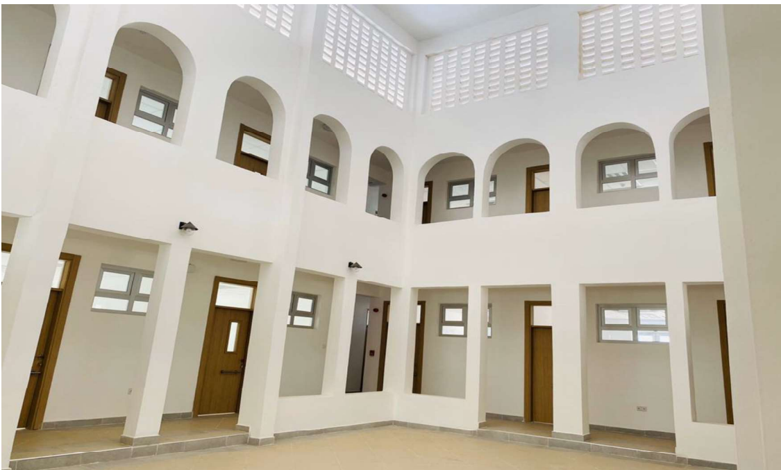
Photos of the EDR building and aerial view of the new NIEC Compound including EDR building.
