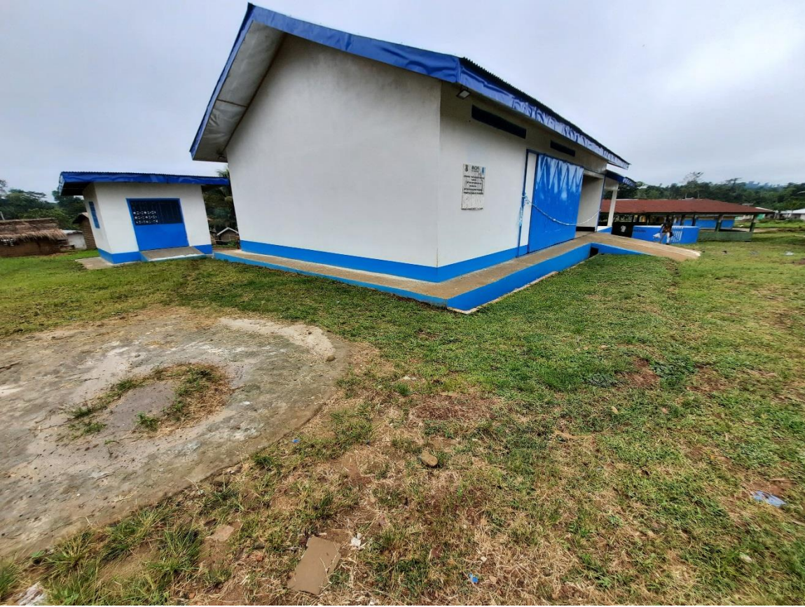
Photo: Newly constructed warehouse in Loguatu
