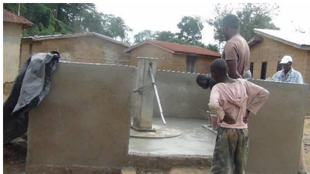
Water drilling pumps renovated by the project
