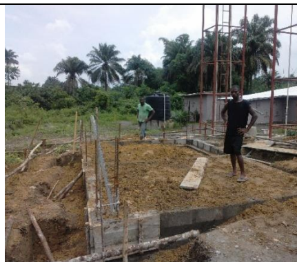
Elevated Water Tower at foundation stage
