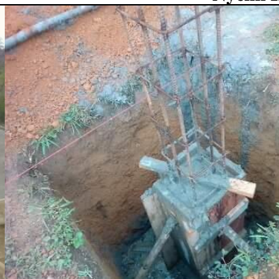
Elevated Water Tower at foundation footing level
