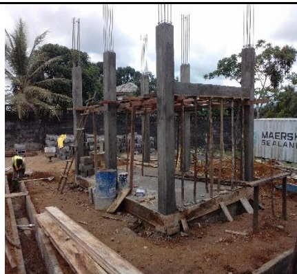
Columns for Elevated water tower
