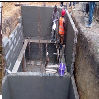
6-Cubicle Latrine Septic tank construction
