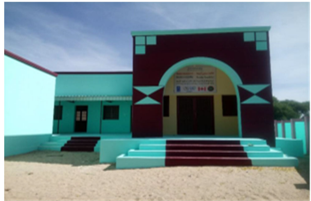
Construction of a Rural Court in Masteri, WD
