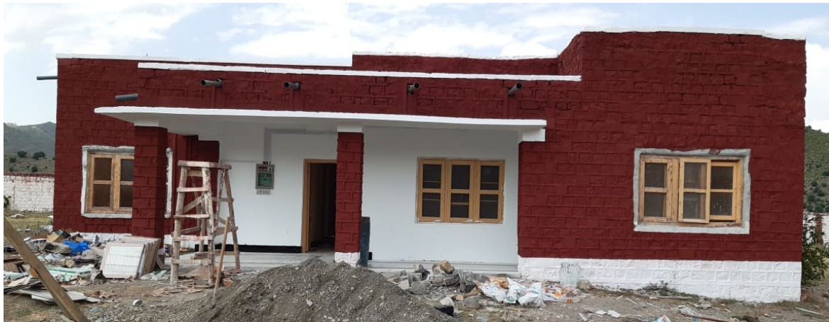
Renovated & refurbished health facility, Civil Hospital Dossali, North Waziristan
