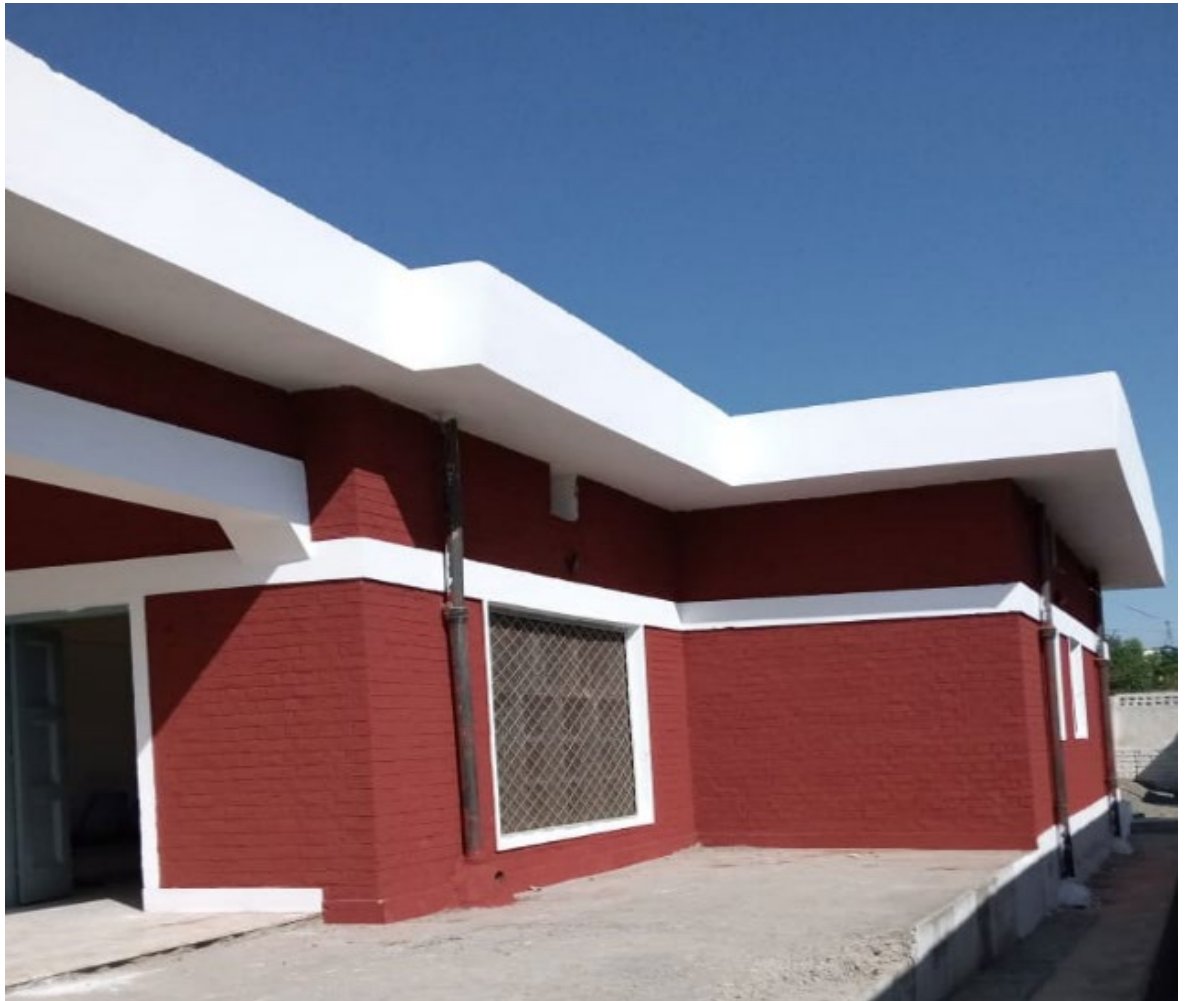
Renovated & refurbished health facility, District Khyber, Civil Hospital Lwara Maina
