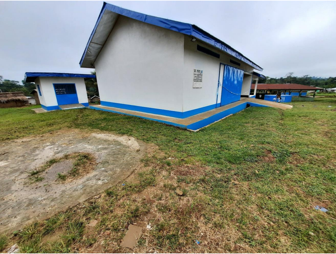
Photo: Newly constructed warehouse in Loguatu
