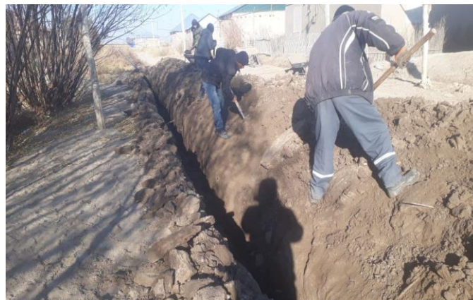
Photos 1 and 2. Reconstruction of the water distribution facility and installation of the water pipeline network at the Beltau Community Centre
