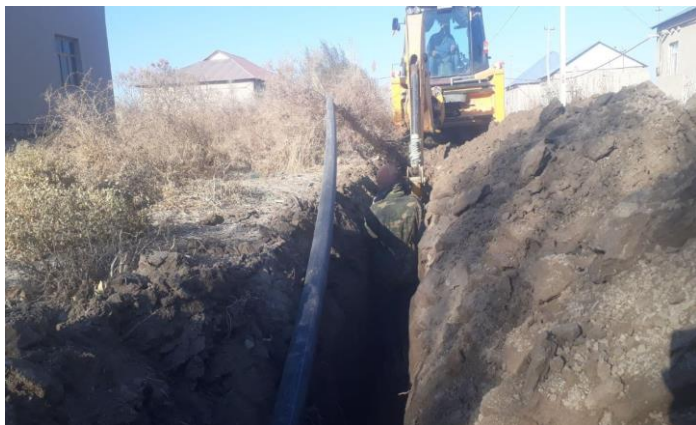
Photos 1 and 2. Reconstruction of the water distribution facility and installation of the water pipeline network at the Beltau Community Centre
