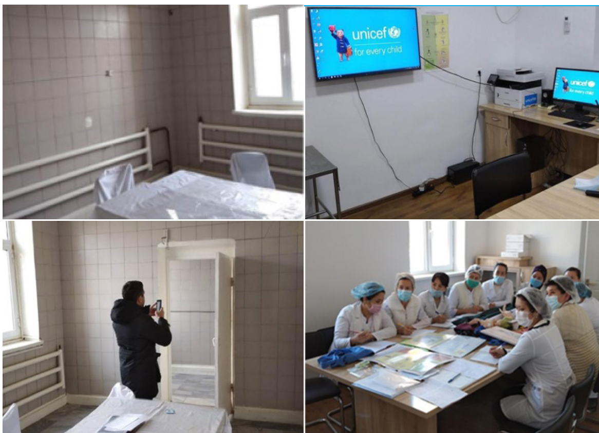
Photo 8, 9, 10 and 11. Before and after renovation of the training room at the Regional Perinatal Center
