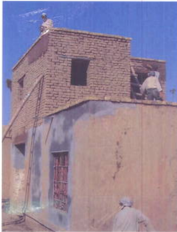
Rehabilitation in progress – detention center guard tower in Mazar-e-Sharif
