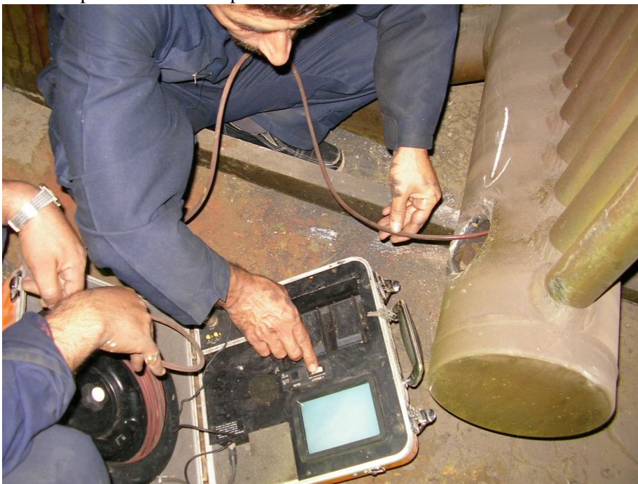
Endoscopic boiler tube inspection
