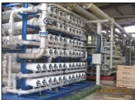
Newly installed RO Skid
