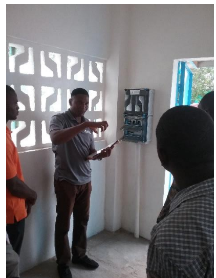
Instillation of control box
