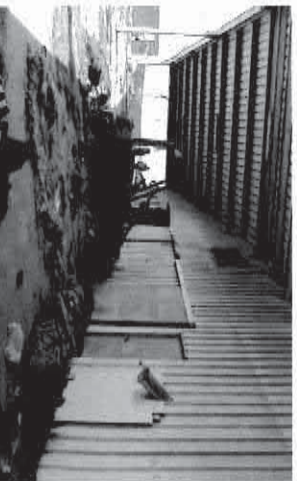
An abandoned fish processing plant in Bosasso to be reclaimed as a training facility.
