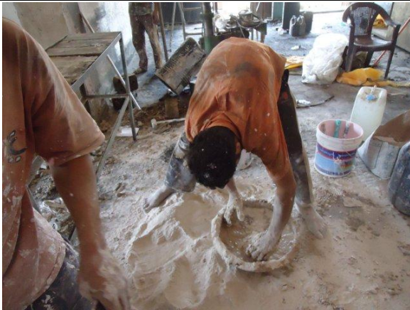
Many resources were used to renovate the workshop.
