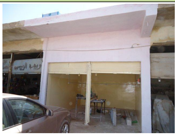
The facade after
