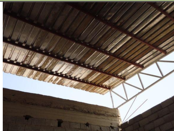
A new shelter was placed above the workshop. 165 m 2 metal shed.
