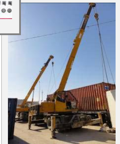
Two 20-tonne cranes offloading container laden with generators, 28 th December 2010
