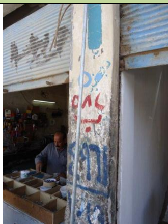
The facade before
