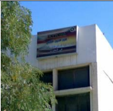
ICTDC centre in Al Atefia near Saif Al Dawla school from outside
