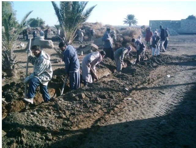
Figure 12 Laying Water Pipelines
