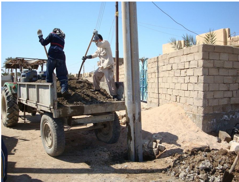
Figure 7: Bringing electricity to the neighborhood
