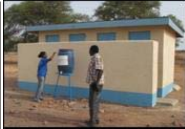
Public latrines built in Twic East County, Warrap State. Photo: UNDP©
