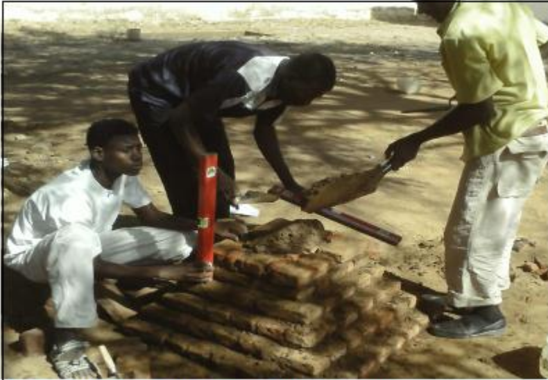
Basic Building Construction Skills Training
